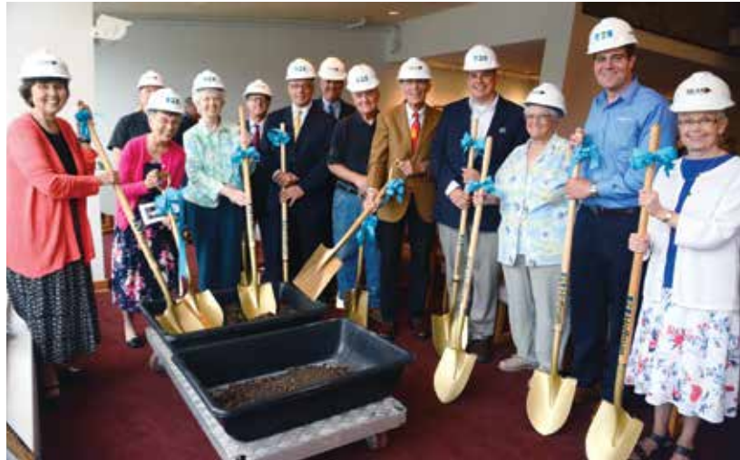
Members of the Congregational Leadership Team, along with staff from our La Grange Park center and representatives from Hoffman Construction Company, put ceremonial shovels in dirt to mark the beginning of construction. Inclement weather prohibited the ceremony from taking place outdoors.
